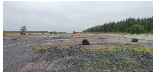
Fig. 26. An image showing the quality of the surface of the track.
