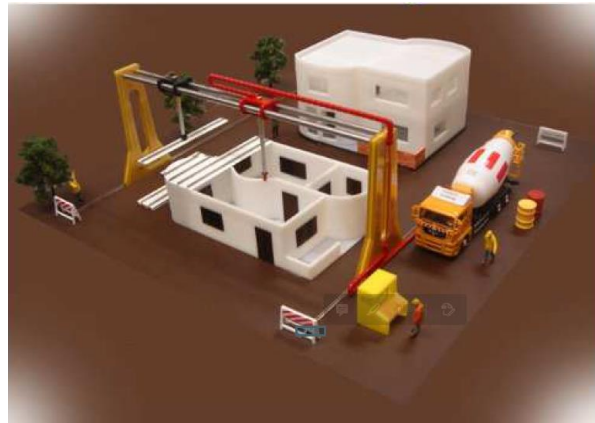
Figure 2 A Cartesian robot assembles prefabricated parts of a house. (Usmanov, et al., 2010, p. 6)
