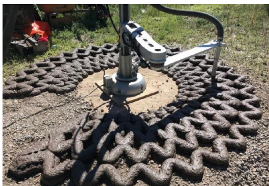
Figure 5. The robot has 2 rotating joints for 2D movement and moves up and down on a pole. (San Fratello & Rael, 2020, p. 27)
