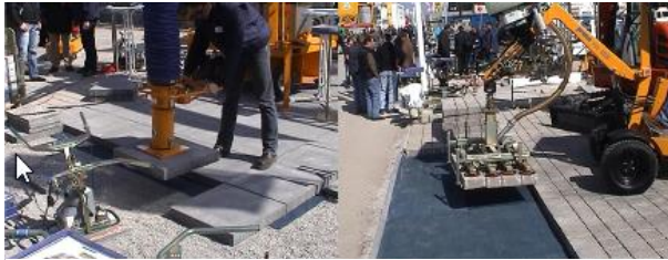
Figure 7. the end effector is made specifically to hold onto the shown bricks to place them without gaps (Vähä, et al., 2013, p. 9)
