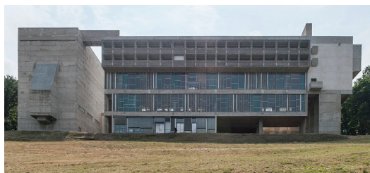
Figure 16: West Façade of the Couvent de La Tourette, showing Xenakis' Stacked Undulating Glass Panels.
