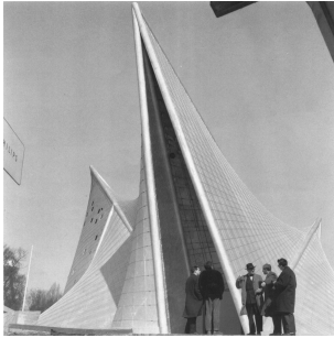
Figure 13: Exterior view of the Philips Pavilion, constructed using ruled surfaces in a similar way to Xenakis's musical glissandi.
