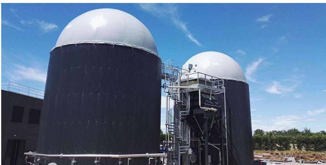
Figure 4: Two Fluence large-scale anaerobic digestion products: EFC digester and sludge digester to treat confectionary wastewater at a facility in Ossona, Italy. Image taken from (Fluence, 2020)
