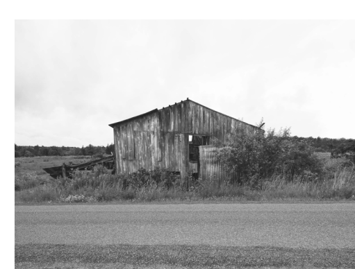
Dilapidated barn sits directly to the road, starting to topple down. The road hides it well.
