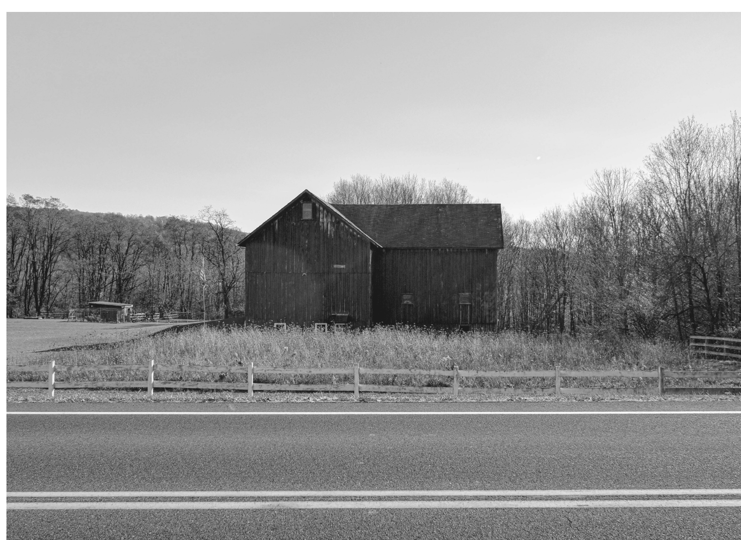
Barn is setback from the road. It sits on a manicured landscape ie: the fence, the field, the mowed grass, the flag.
