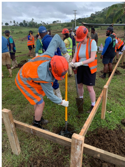
Figure XXXVIII - Digging the Foundations
