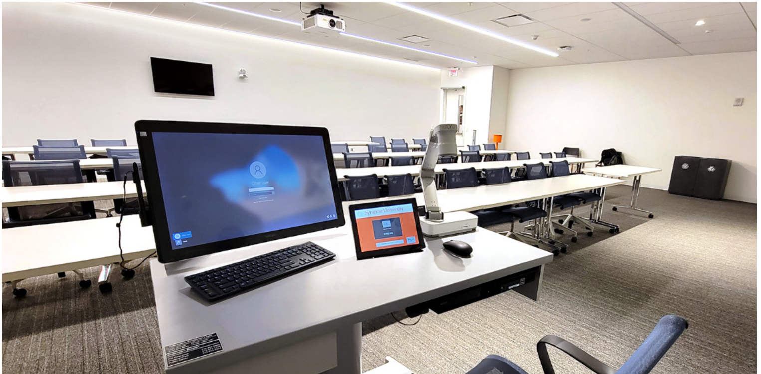
The standard classroom presentation workstation is a Steelcase AirTouch height-adjustable table outfitted with a micro-PC, an annotation touch screen, a Blu-ray® player, a document camera, AV connectivity with power, and an Extron TLP Pro 1025T 10" Tabletop TouchLink Pro Touchpanel for system control.
