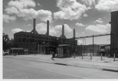
C2 Case Study No. 2 Walkerville Industrial Corridor
