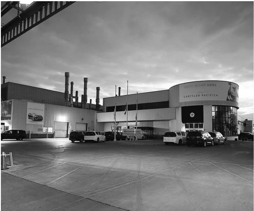
The current main entrance is shown vacant in November 2021 / Dan Janisse, Windsor Star.
