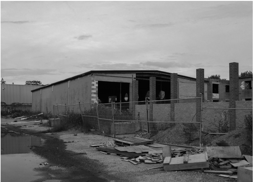
One of many abandoned industrial lots along McDougall Street, 2023 / Photo by Author
