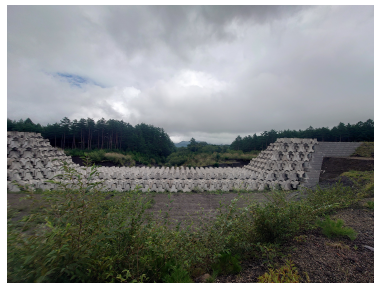
Figure 16: Sabou - Dam to prevent landslides
