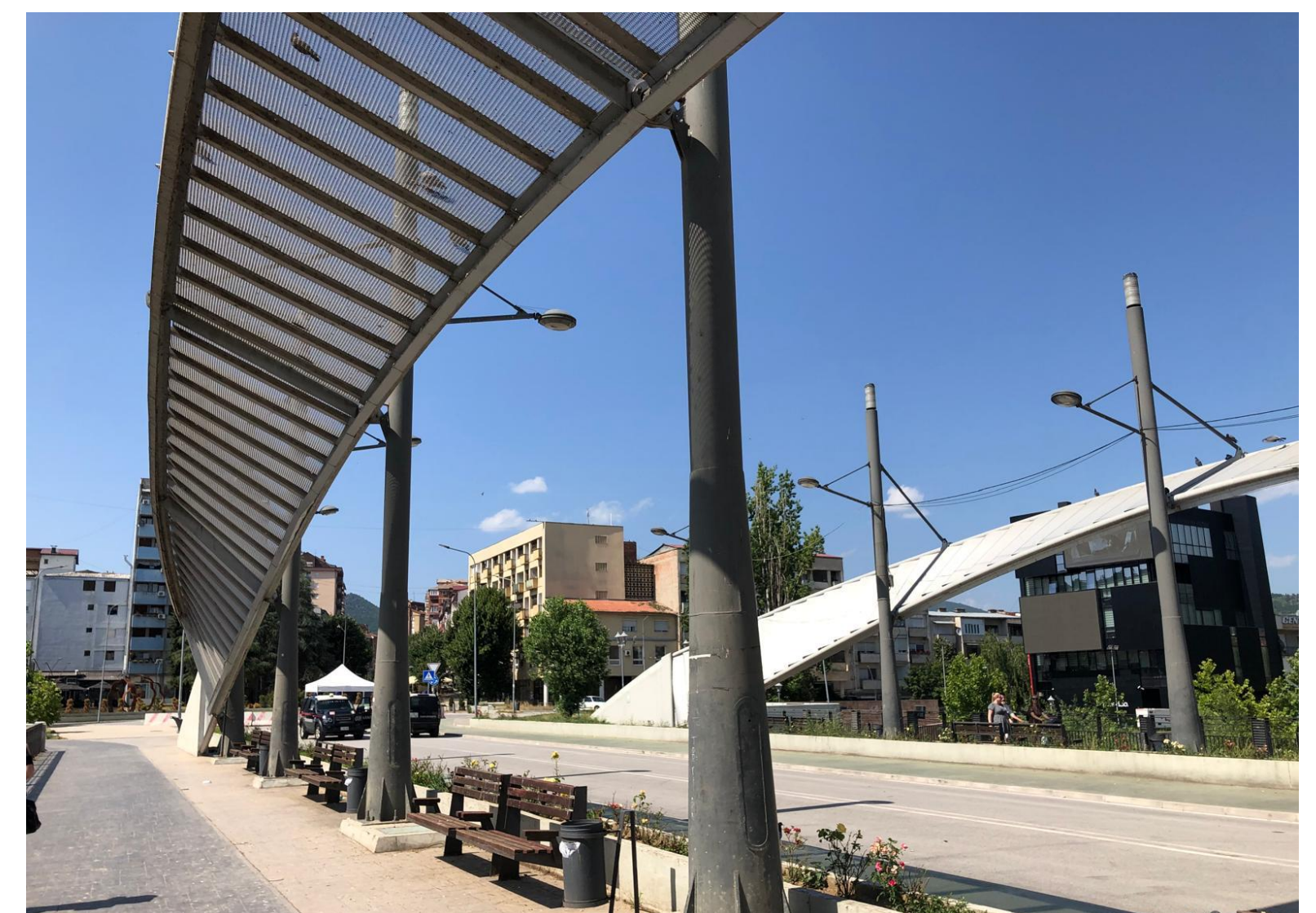
Figures 3 & 4: Photos from the main bridge in Mitrovica that divides majority ethnic Serb North Mitrovica and northern Kosovo from majority ethnic Albanian South Mitrovica and the rest of Kosovo.
