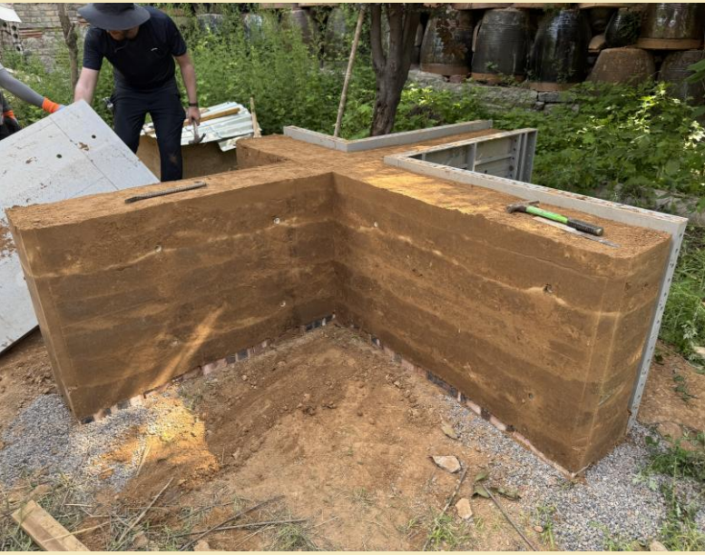
Rammed-earth test wall
